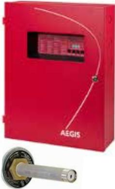
HP CO<sub>2</sub> fire suppression systems are designed to minimize the impact from a fire to the collector and to the surrounding area. The HP CO<sub>2</sub> fire suppression system follows the design practices in NFPA 12, which calls for the flooding of a collector with CO<sub>2</sub> to a 75% concentration. The HP CO<sub>2</sub> fire suppression system typically uses one, two or three CO<sub>2</sub> cylinders piped to a discharge nozzle mounted in the collector or the inlet duct.
